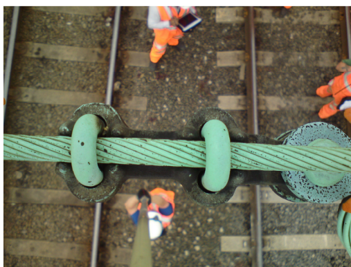
Figure 6 – Example wire inspection image*
